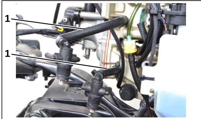
1. Drain valve hoses
