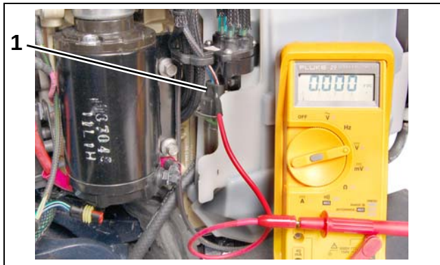
1. Oil injection pump electrical connector
